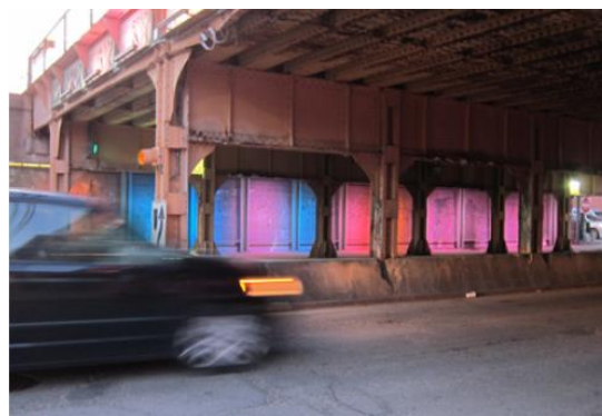
Figure 6. Existing Conditions Oak Park Avenue Viaduct – North Side Facing Southeast
