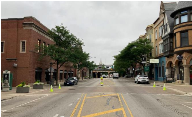
Figure 1. Existing Conditions Oak Park Avenue Facing South Towards North Boulevard
